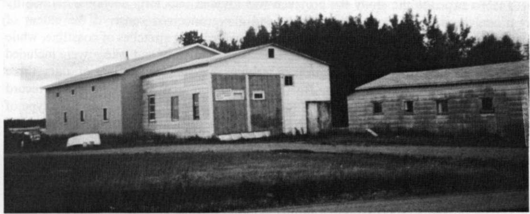
Figure 2: The late Robert F. MacPherson's boatshop, west of Wallace, Cumberland Country, is an example of an expansion to accommodate the ever-increasing size of fishing boats. On the right is the original shop. The larger shop built to replace it has been expanded.
