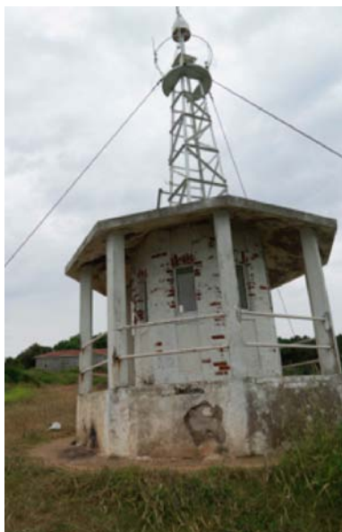
Watch tower base
