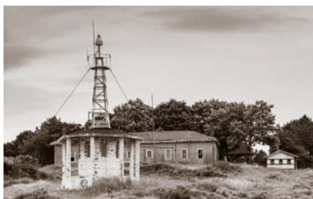
Watch tower base with refuge house behind
