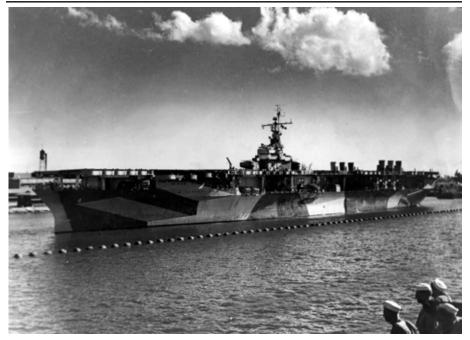
USS *Ranger* after its partial modernization during May to June 1944. Visible is its new radar suite composed of an SM height-finder radar and an SC search radar. The 5"/25 battery was removed as weight compensation for the strengthened flight deck, deck catapult, new radars, and new combat information center (CIC). (NHHC)
