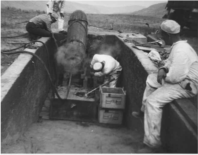
One of the two Esquimalt mines at the end of being steamed out on 29 or 30 May 1952. This photograph shows more details of the process, including the large container used to receive the melted explosive, and the boxes (right) used to haul it away for burning. (Credit: © Government of Canada. Reproduced with the permission of Library and Archives Canada (2023). Library and Archives Canada, Department of National Defence fonds, E-19108-1)
